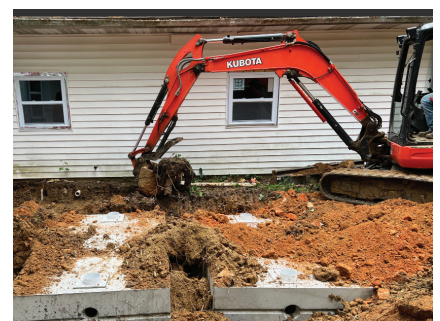
New septic tanks delivered this past week.
